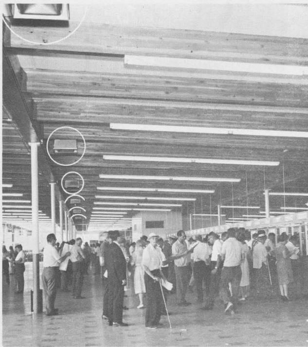
Center Section of Grandstand Mezzanine
